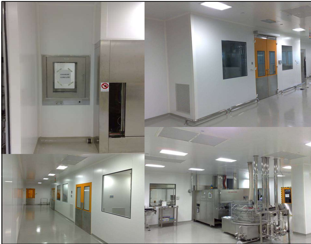
Figure 14: GPM50 Systems Setup
