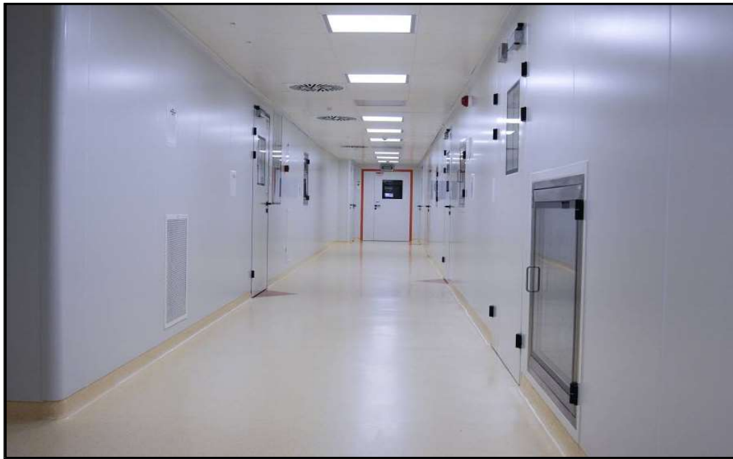
Figure 12: GPM50 System Finishing After Completed
