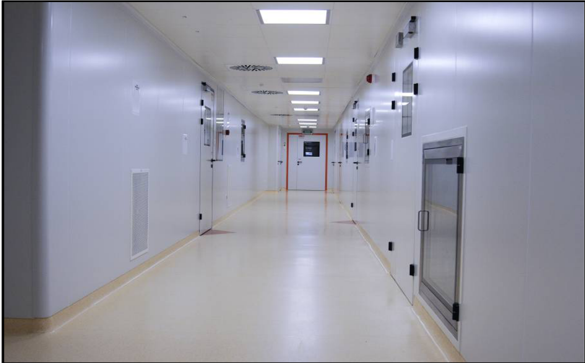
Figure 12: GMP50 System Finishing After Completed
